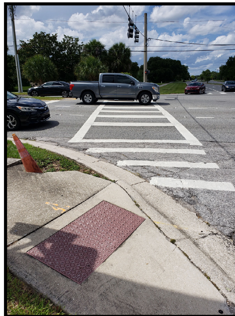
Damaged Crosswalk at SW corner of Central Florida Pkwy. & Gateway Ave. with Ped ramp connecting to one direction
