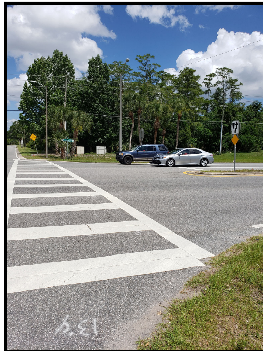
South crosswalk at Orangewood Blvd. & Gateway Ave. showing no connection to sidewalk
