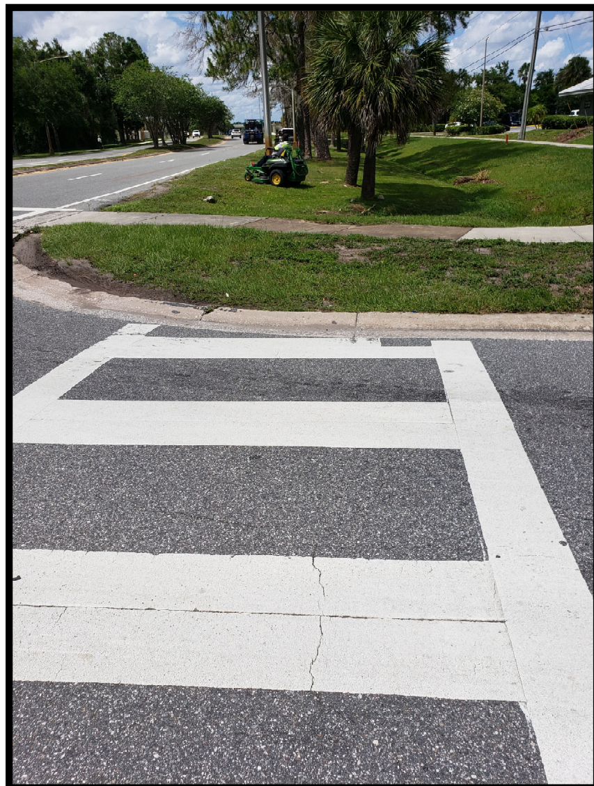
East crosswalk at Orangewood Blvd. & Gateway Ave. showing no curb ramp in NE corner
