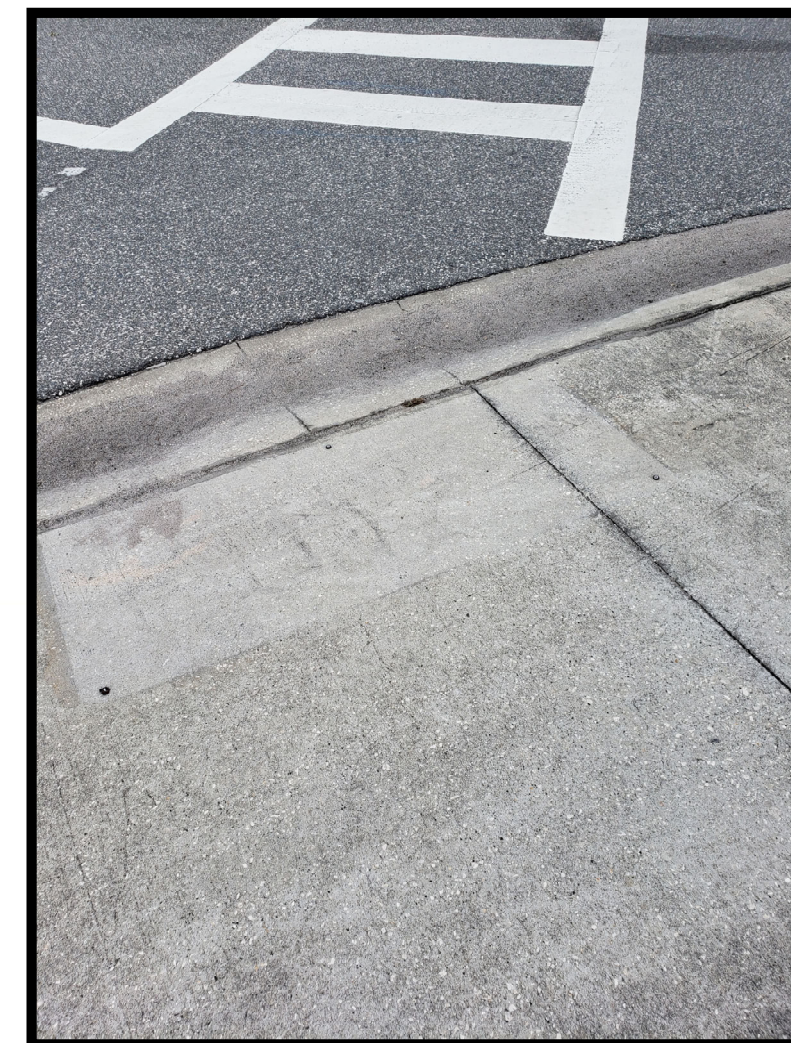
Missing Detectible Warning Strip at SW corner of Central Florida Pkwy. & Oranewood Blvd.
