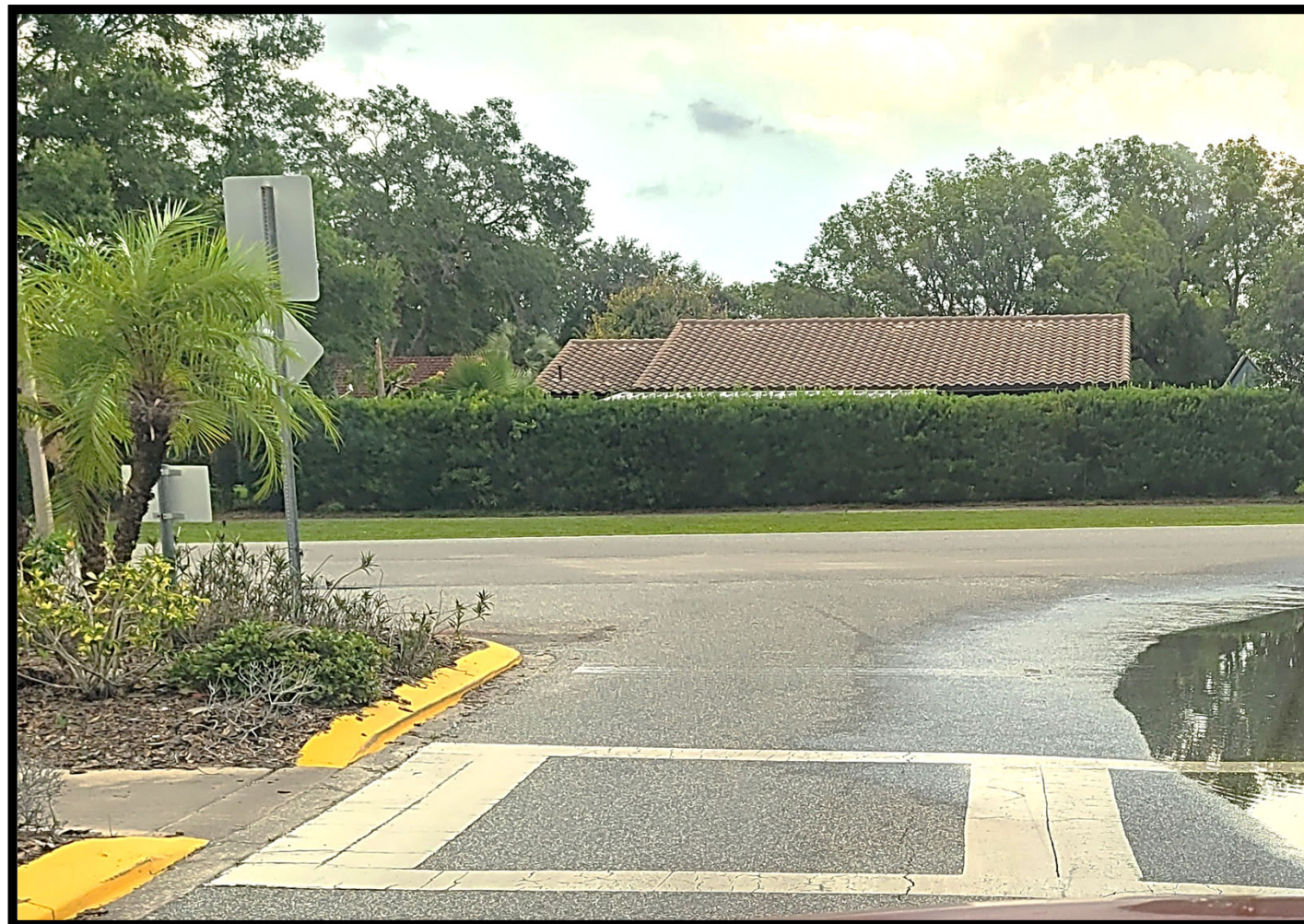
Flooding at Gateway Avenue & Marco Polo Drive with Clogged Ditch Bottom Inlet
