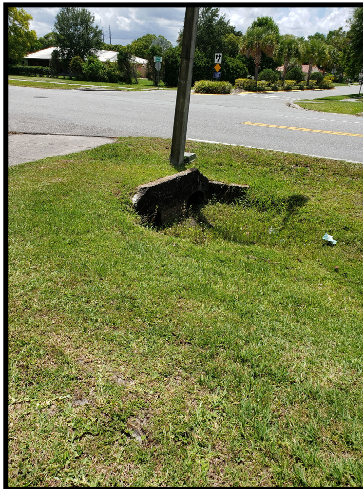
Gateway Avenue & Wildflower Road with Clogged Drainage Pipes
