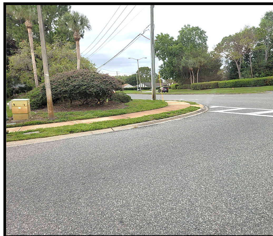
Poor Sight Distance Looking Left at Orangewood Blvd & Deer Creek Drive (EB)
