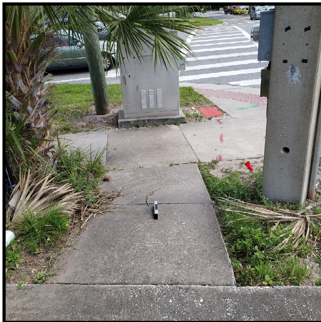
Crosswalk at NE corner of Central Florida Pkwy. & Gateway Ave. with steep slope ending at signal cabinet
