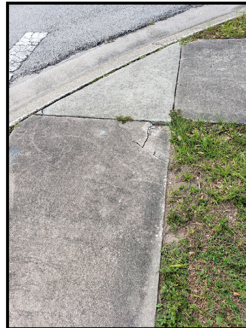
Sidewalk at Gateway Ave. & Larissa St. with no sufficient flat landing area
