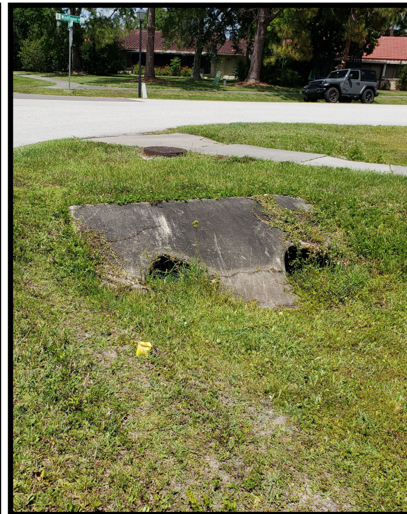
Gateway Avenue & Wildflower Road with Clogged Drainage Pipes
